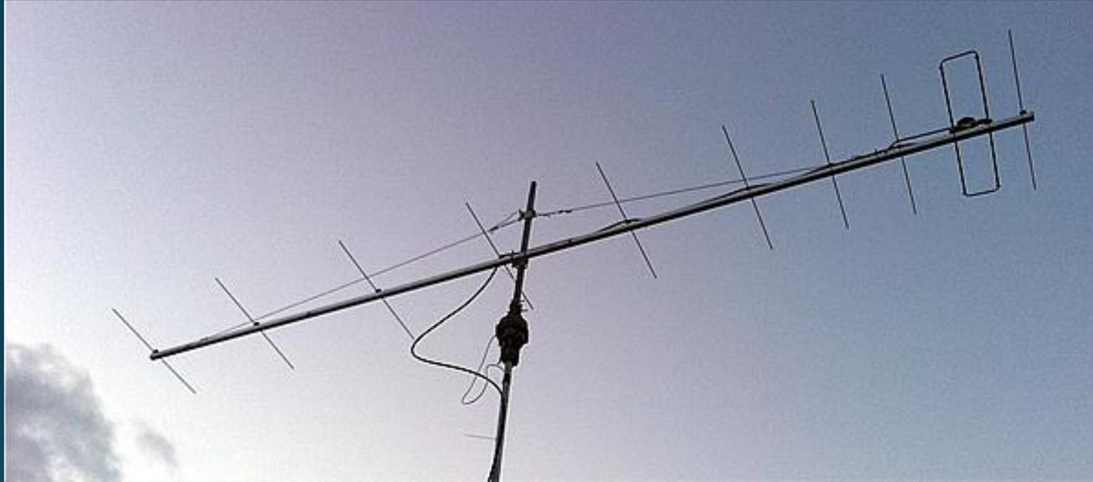
**Back Brace center is too close to boom; a tight pull on cables will put boom into severe compression.**
