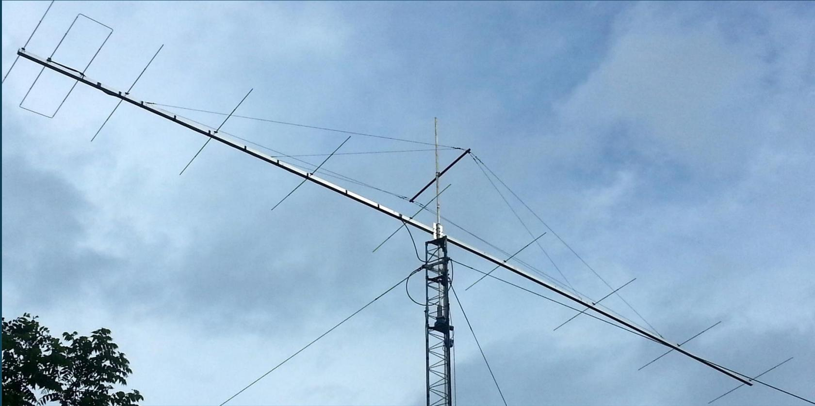
**Nice upper double boom truss: Cross bar is high enough and wide enough to create good pulling geometry. Intermediate boom guys provide additional tweaking of boom straightness.**
